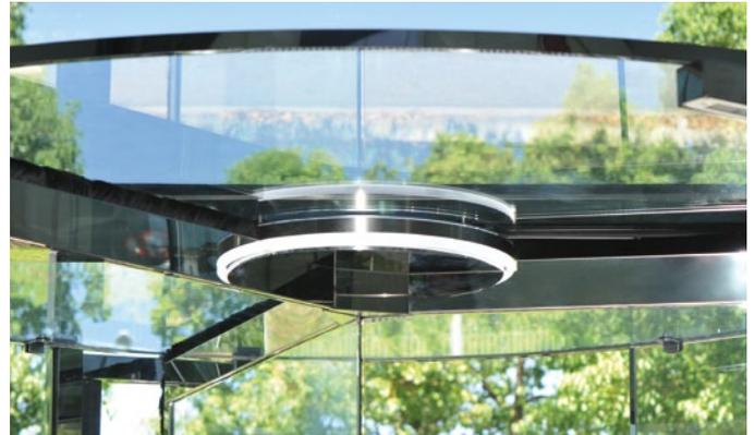
This is the first time that the new drive technology has made it possible to combine the elegance of a slim glass ceiling construction with a drive system concealed in the ceiling - even in a fully automatic version.
