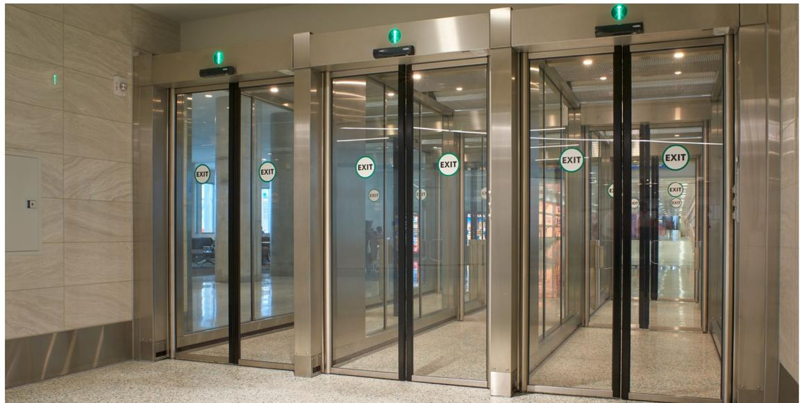
ELBC technology employs real-time video analytics, 3-D imaging, system monitors and motion sensors that integrate with airport security and fire detection systems. dormakaba's exit lane breach controls sophisticated "smart technology" detects and identifies suspect persons and objects left unattended, and thrown objects, while greatly
