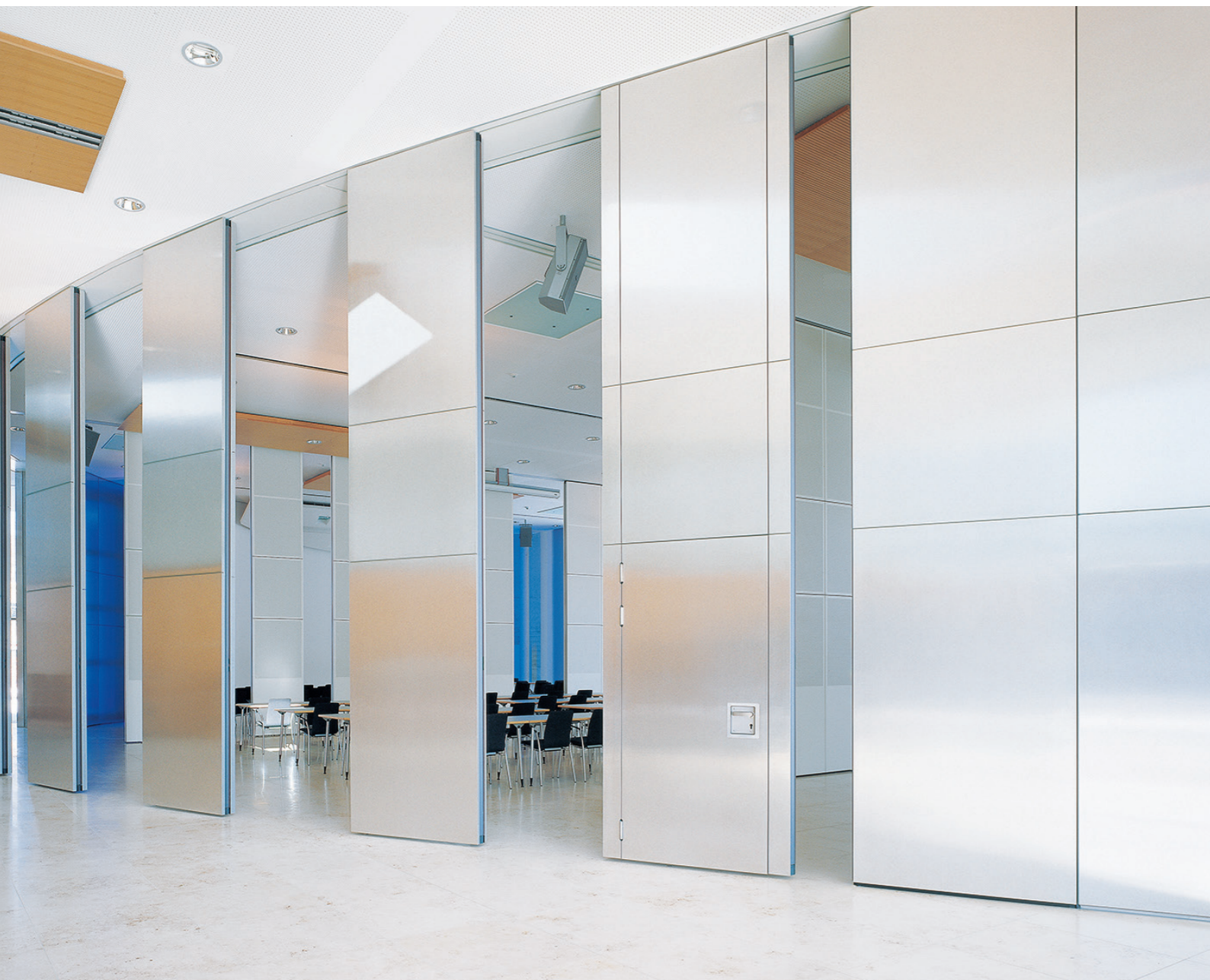
Progetto: WMF Communication Center, Geislingen an der Steige, Germania
