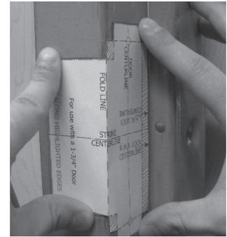
2. Peel adhesive backing and paste the folded template square to the frame.
