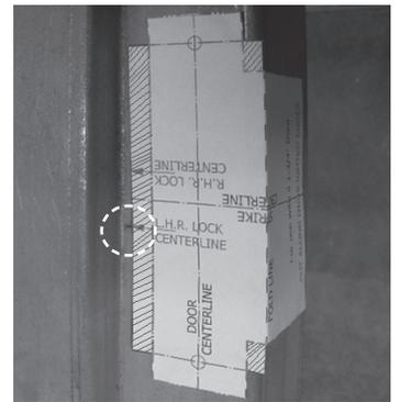
**3.** Carefully cut the frame inside the un-shaded area marked on the template.
