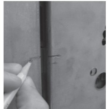
**2.** Horizontally align the proper Template Lock Centerline with the Lock Body Centerline marked on the frame. Peel adhesive backing and paste the folded template square to the frame.
