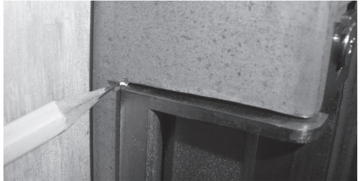
3. Peel the adhesive backing from tape on the back side of the appropriate faceplate. Remove the strike mounting screws. Hold the strike in position as marked on frame. Carefully position the faceplate onto the strike and secure to the frame.
